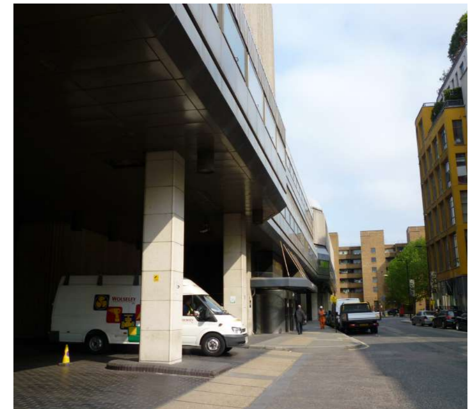
Fig 2.5 Sampson House - Service Yard
