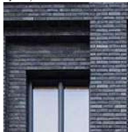
Fig 7.77 light blue / grey brickwork
