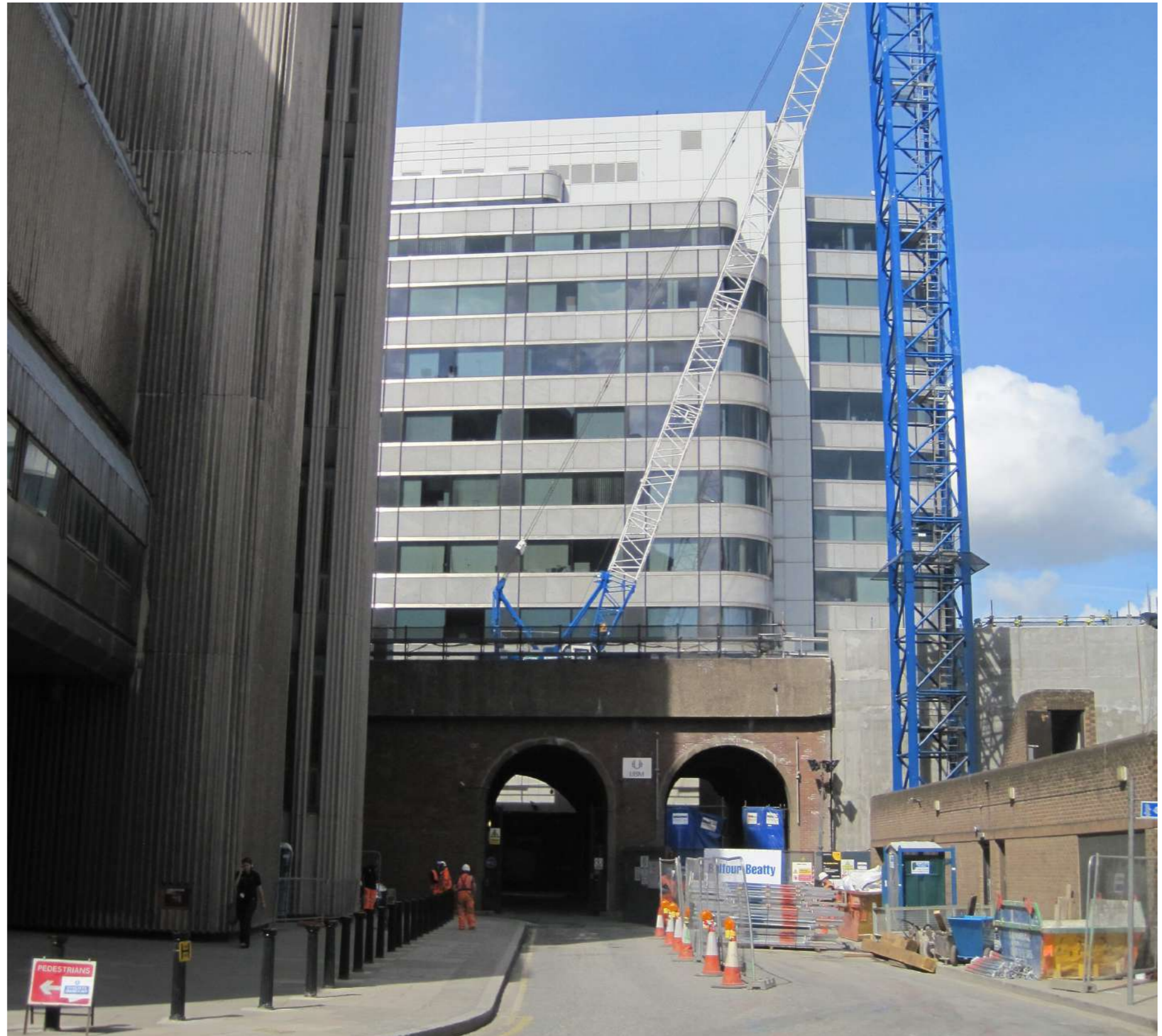
Fig 5.5 Existing View looking West from Hopton Street (Northern end).
