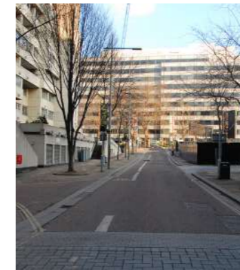
Fig 1.25 Existing wall at end of Upper Ground
