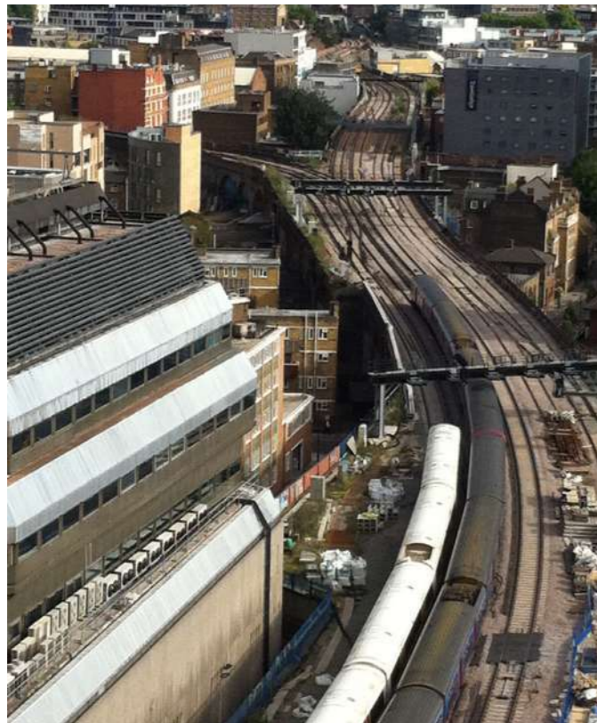
Fig 1.3 Thameslink viaduct looking south
