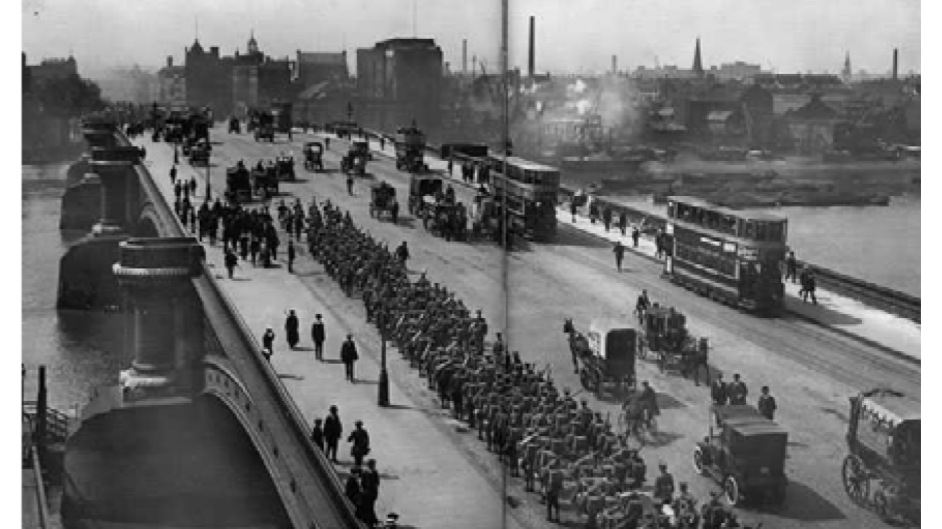
Fig 1.8 Blackfriars Bridge circa 1890
