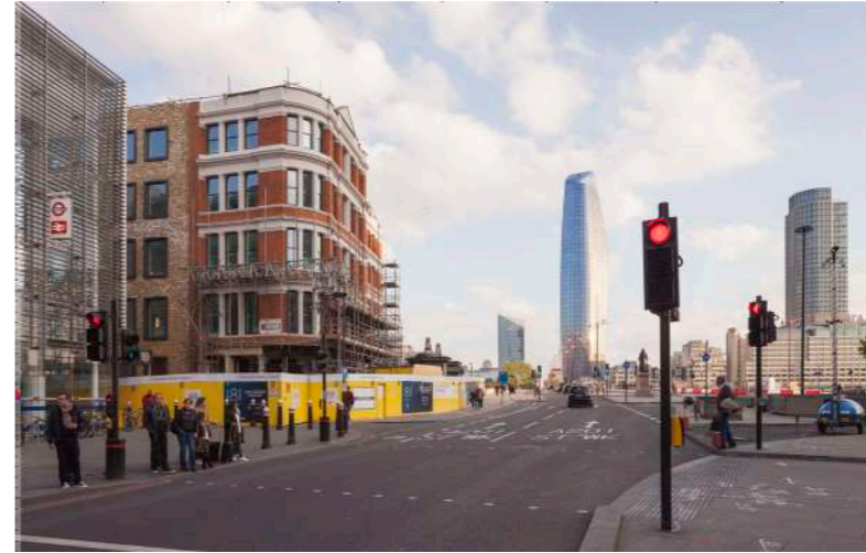
Fig 3.25 IL22 - Blackfriars Bridge northern end
