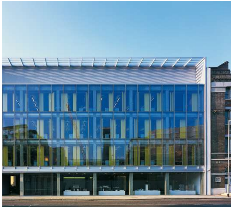
Fig 1.55 85 Southwark Street - Office
