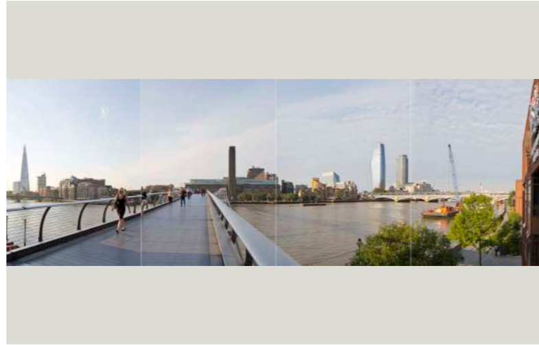
Fig 3.24 IL21 - North side of Millennium Bridge (panorama)
