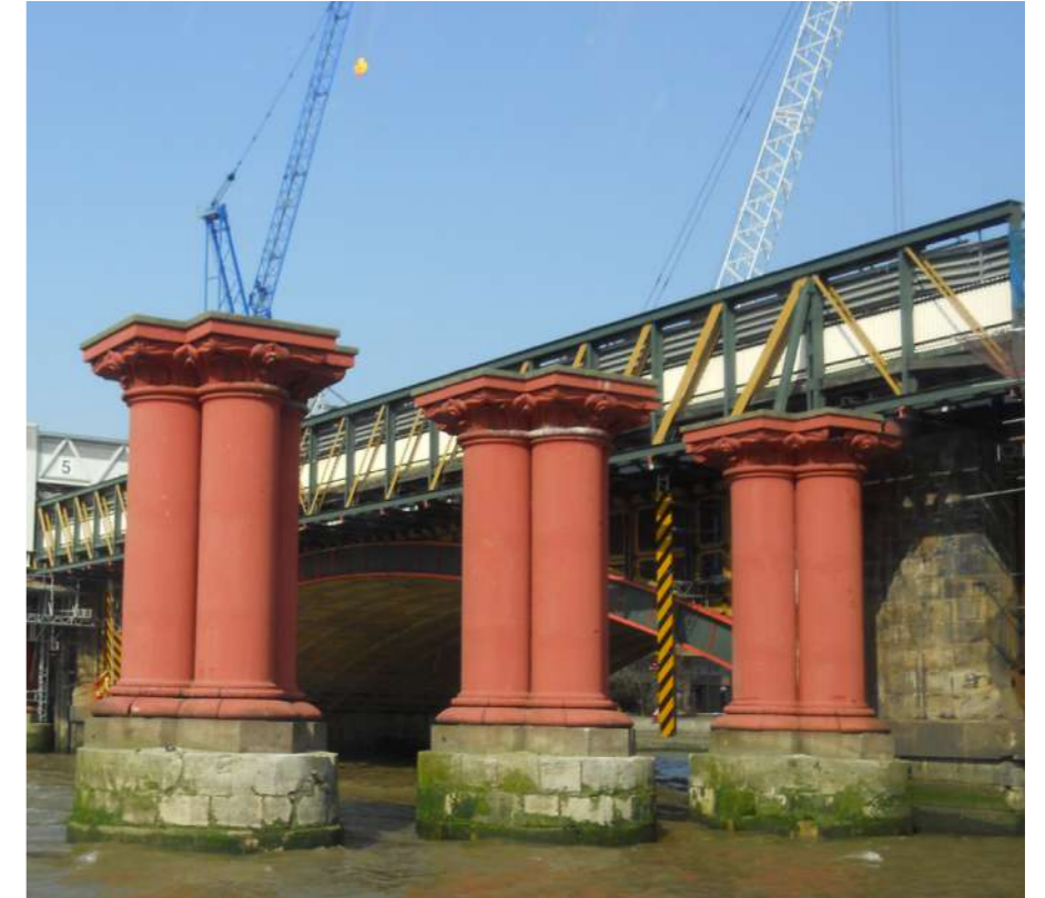
Fig 1.17 Southern Abutment to former West Blackfriars and St. Paul's Rails Bridge
