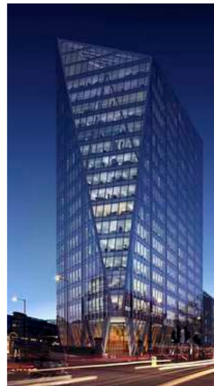
Fig 1.53 231-241 Blackfriars Road - Office Development
