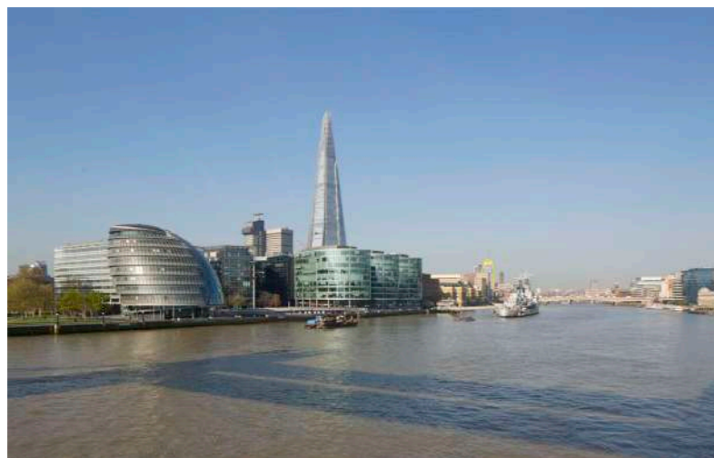
Fig 3.10 LVMF 10A.1 - Tower Bridge: upstream - the North Bastion
