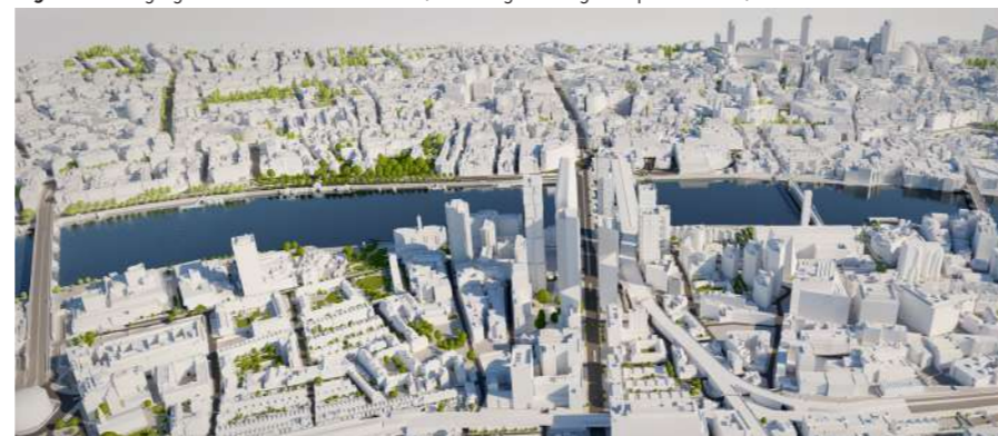
Fig 5.29 Existing Aerial View from South (including existing Sampson House)
