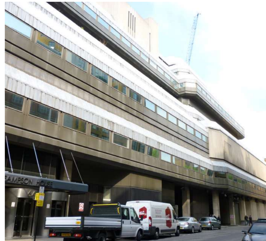
Fig 4.11 Poor public realm in the existing condition
