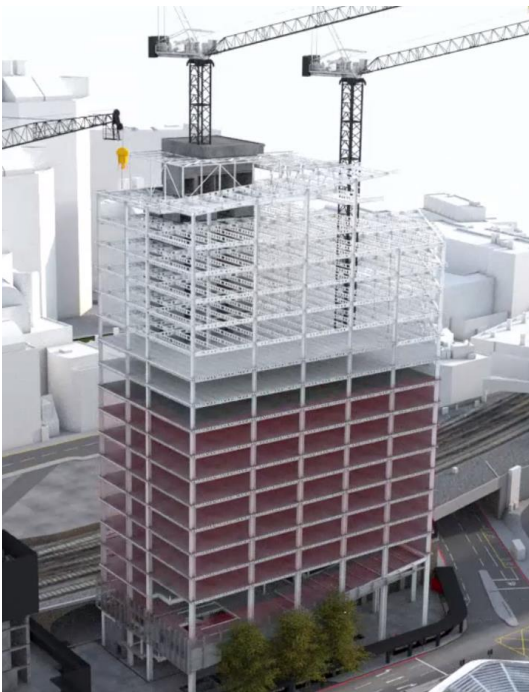
Figure 19 Snapshot from our animation detailing steel frame progression
