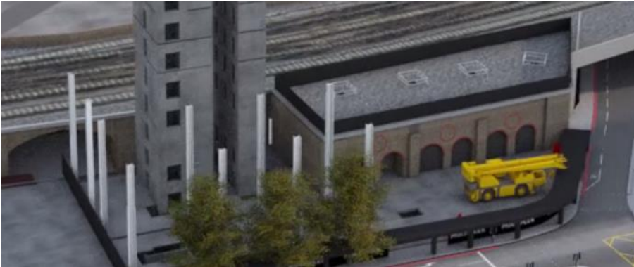
Figure 15 Mobile crane approximate position for column installation
