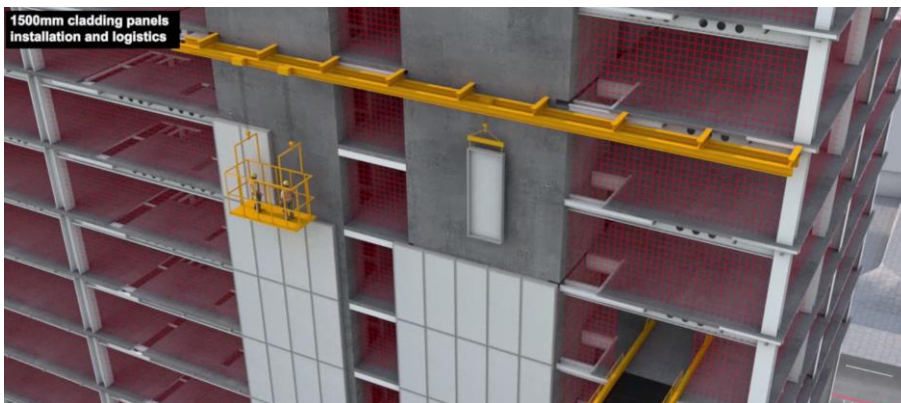
Figure 22 Double monorail installation technique
