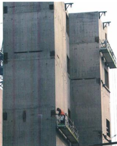
Figure 14 Image showing a cradle for fin plate install
