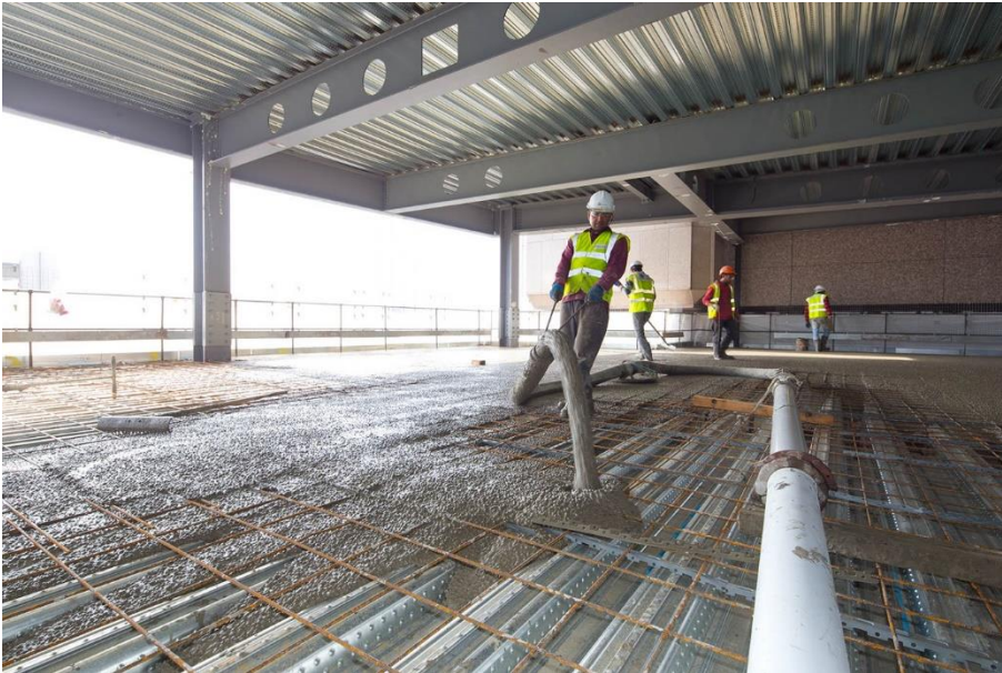
Figure 18 An image showing concrete being pumped on metal decking
